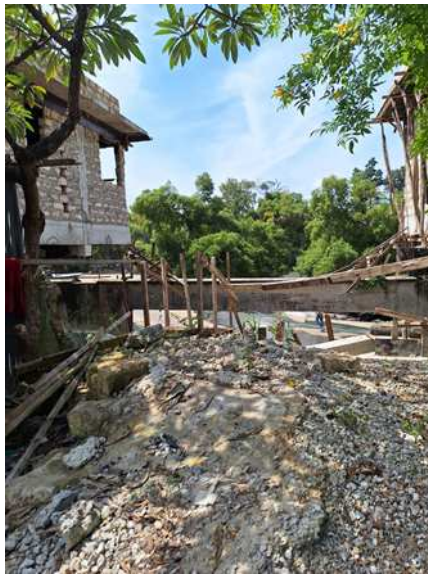
c. The construction on the site
